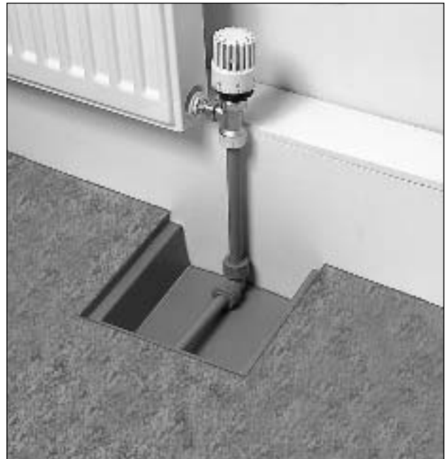
Figure 3 Installation in a suspended floor (all dimensions in mm)
