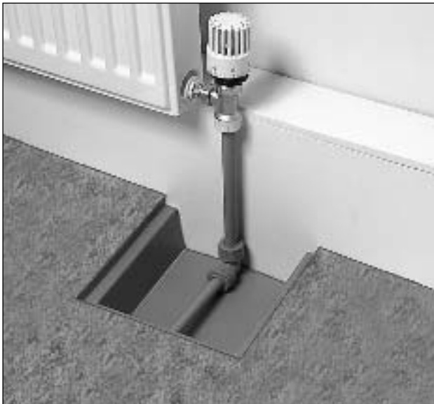
Figure 3 Installation in a suspended floor
