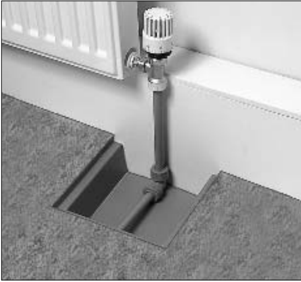
Figure 3 Installation in a suspended floor
